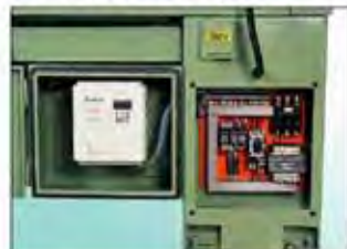
▲ Electrical box for slant head Lathe
